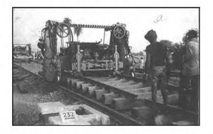
Fig. 15.4 (a) Portal cranes laying concrete sleeper
