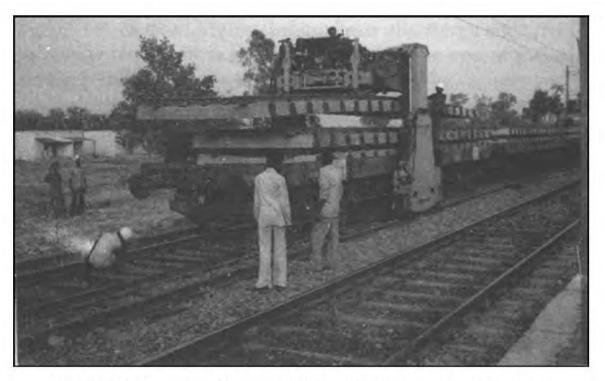
Fig. 15.4 (b) Portal crane licking up concrete sleeper panel
