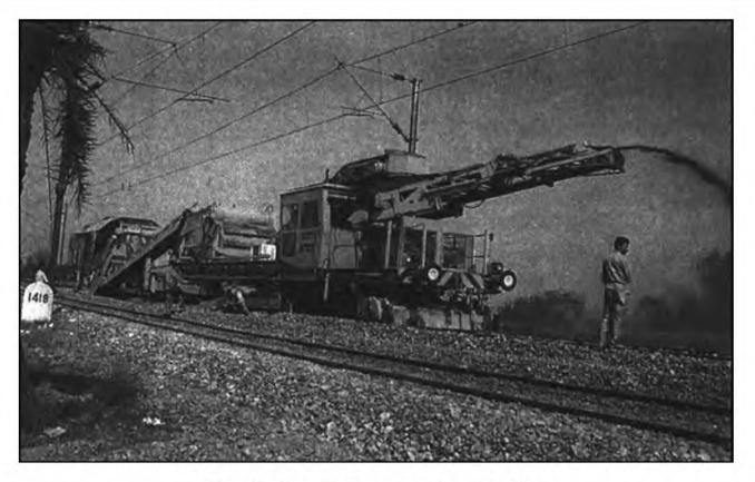
Fig. 12.12 Ballast cleaning machine
