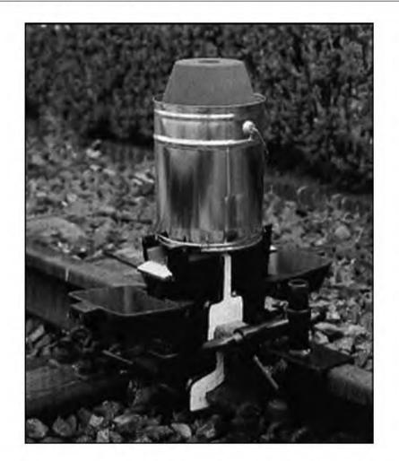
Fig. 9.3 A Single Use Crucible (See also Color Plate 3)
