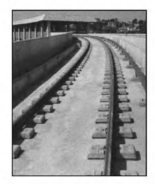
Fig. 18.5 Low vibration track (See also Color Plate 15)
