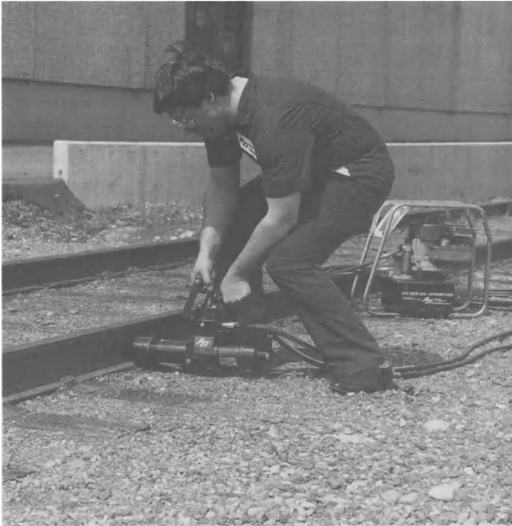
Figure 7 RailTec System In Use On Existing Track
