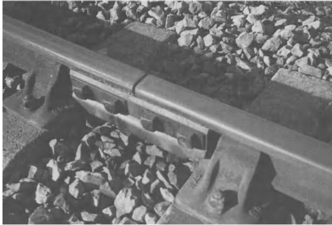
Figure 1 Typical Bolted Rail Joint
